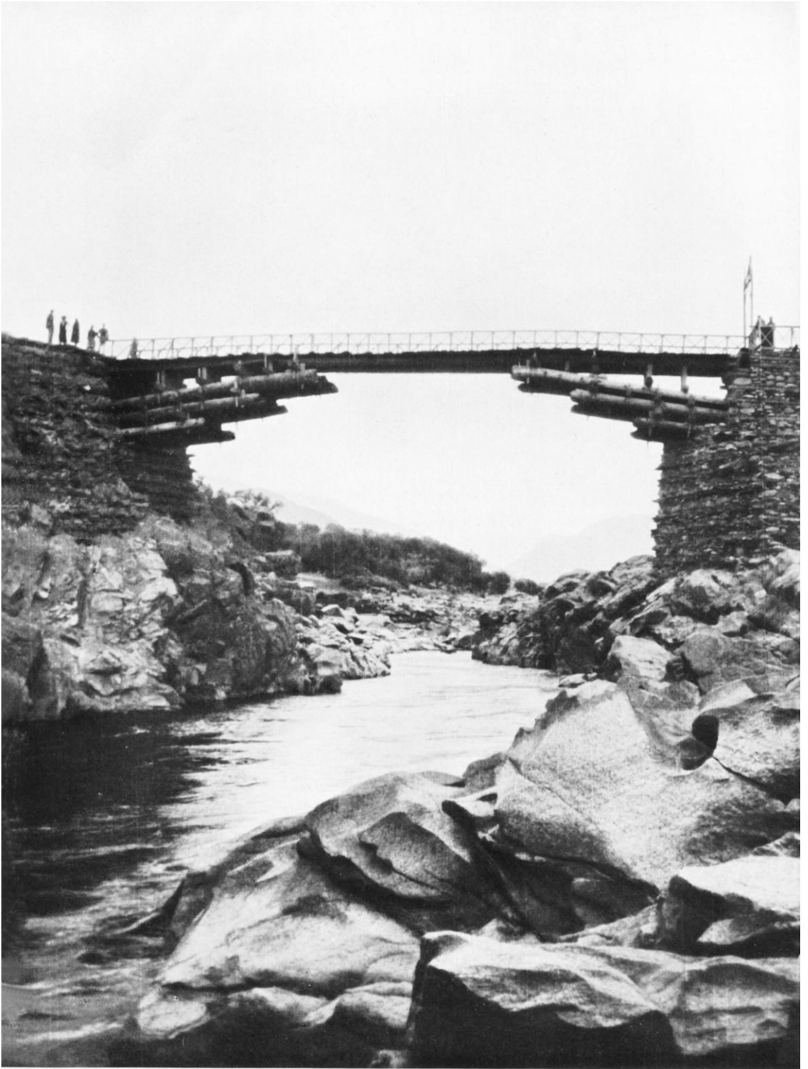
Bridge over the Swat river at Paiti
